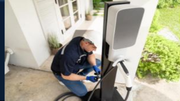
Pemasangan Charging Station Mobil Listrik
